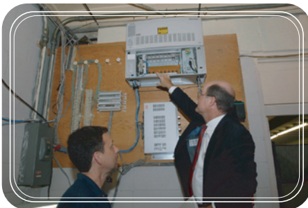
Greg McConnell of Louisiana Office Supply (left) and Richard Peak of Preferred Telephone designed a Toshiba Strata CIX system with battery backup so the system stays live even with power surges and outages.
